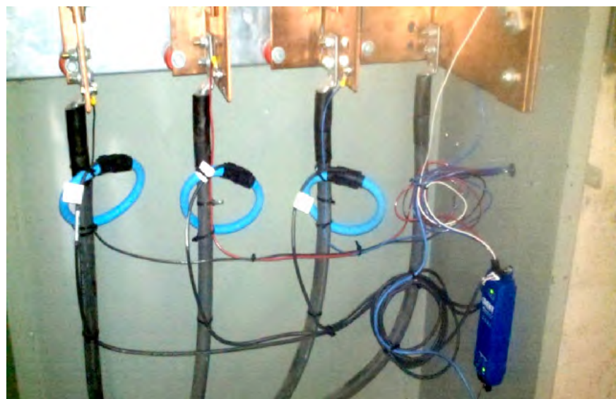
Figure 2b: The PowerScout senses current and voltage flow in the supply lines at Storage Post in Long Island City, New York.
