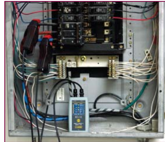
L102 recording two phases of primary feed.
