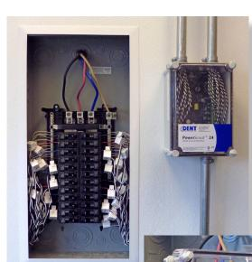
Right: The PowerScout is line powered and the broadband power supply accommodates voltages from 80-600VAC
